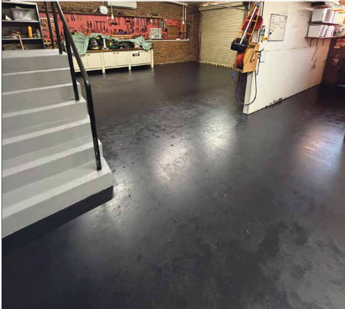
The shiny resurfaced Men's Shed floor.
