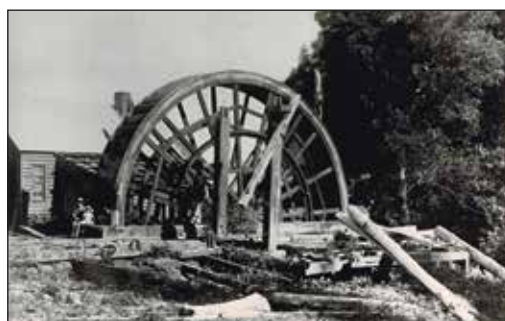
The undershot waterwheel of Christian and Campey's sawmill.
