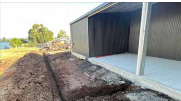
Drainage works underway as the New Gisborne Scout Hut nears completion.
