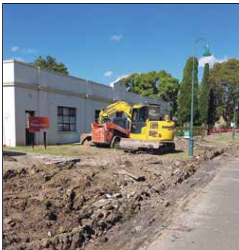
The footpath and gutters between the library and the old courthouse in Hamilton Street are being replaced.
