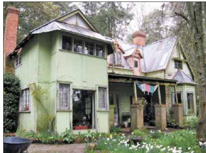
Fontainebleau sadly dilapidated in 2015. Picture Volker Janssen
