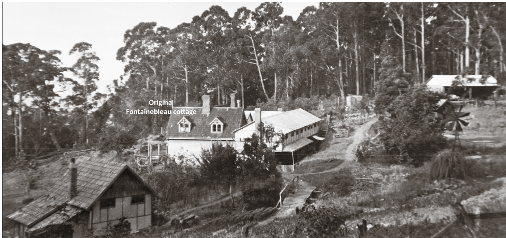
Fontainebleau, Mount Macedon, c1920s, showing later addition for guest house accommodation.
